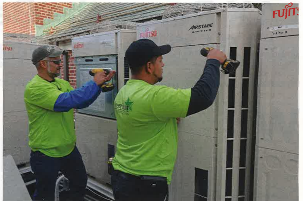
ALL SYSTEMS GO: Hector Pacheco (left) and Sergio Molina (right) close up Airstage VRF units after servicing the units for the first time.
