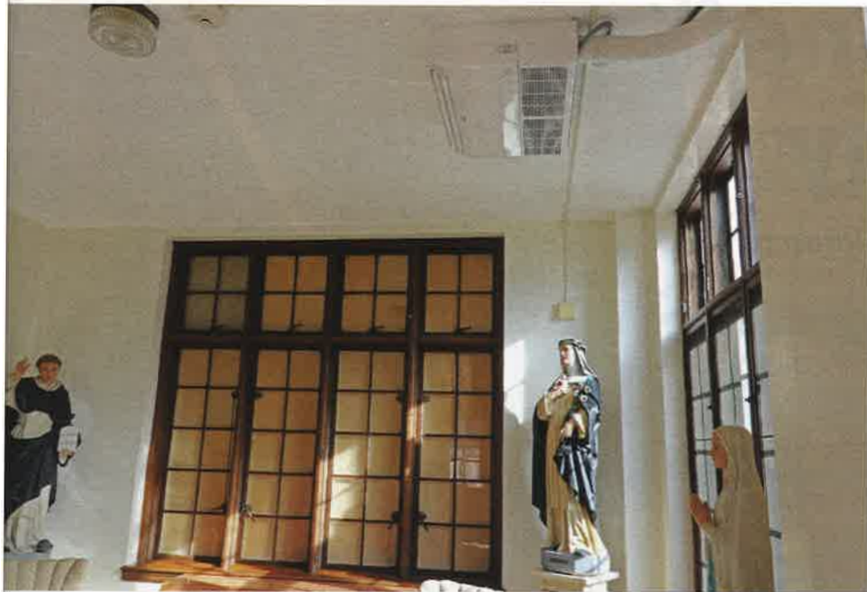
NEW AND IMPROVED: The new VRF system uses a wide variety of indoor units to serve different spaces.
