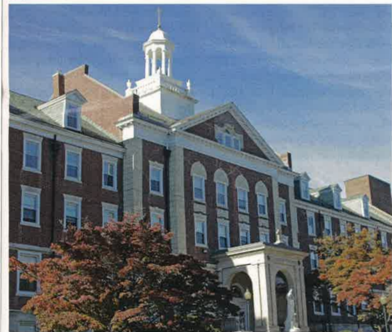
ANTIQUATED APPROACH: The 100-year-old Convent of St. Dominic was previously heated with a steam system and used window units for cooling.
